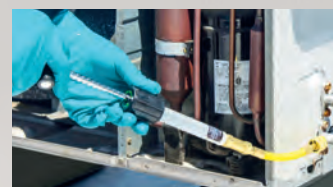
Inject dye with a turn of the handle.
