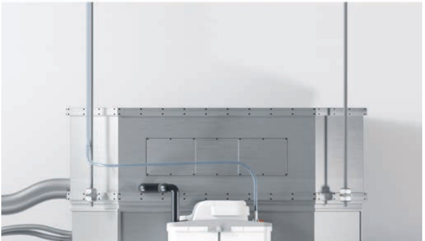
Max Hi-Flow screw mounted to cassette unit
